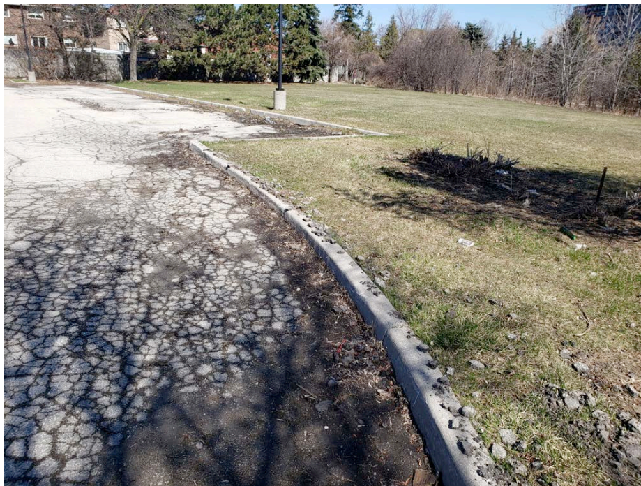
Photo 9: Northeast side of the study area west side. View to the northwest.
