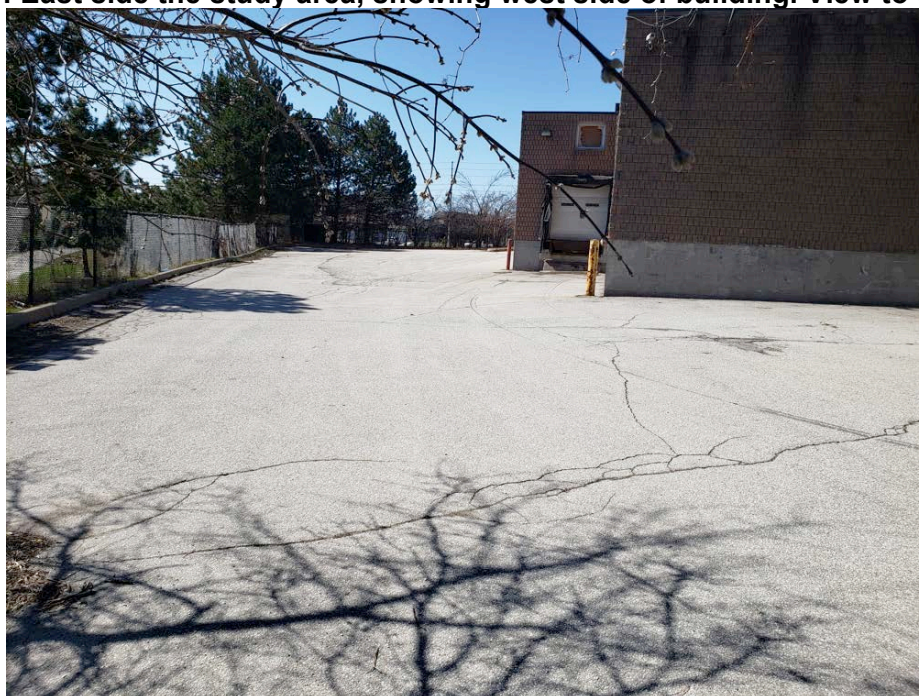
Photo 12: East side the study area, showing northeast side of building. View to the south.
