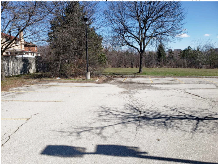
Photo 4: Northwest corner of the study area west side. View to the north.
