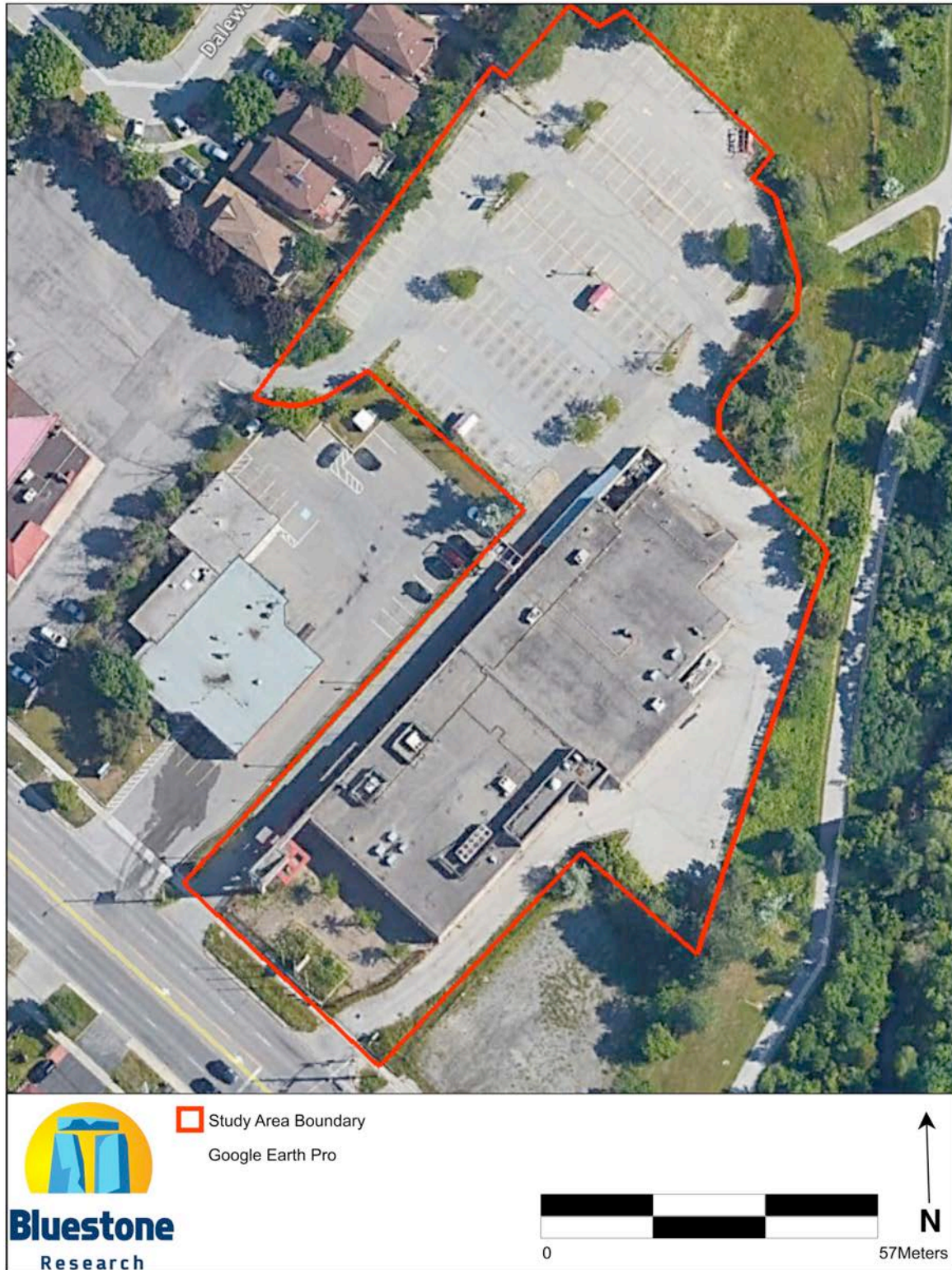
Figure 2: Air Photo Showing Study Area
